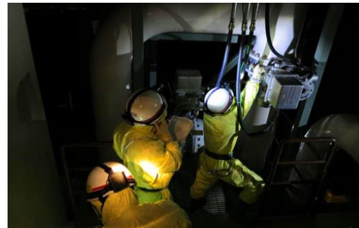
Drills opening valves used in containment vessel vents (Chubu Electric Power website)
