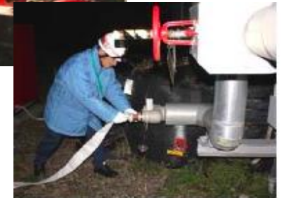
Drills for injecting water to reactors/spent fuel pools (Tokyo Electric Power website)
