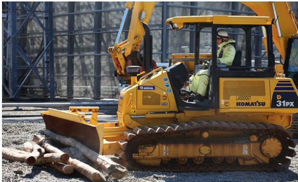
Debris removal drills (Chubu Electric Power website)
